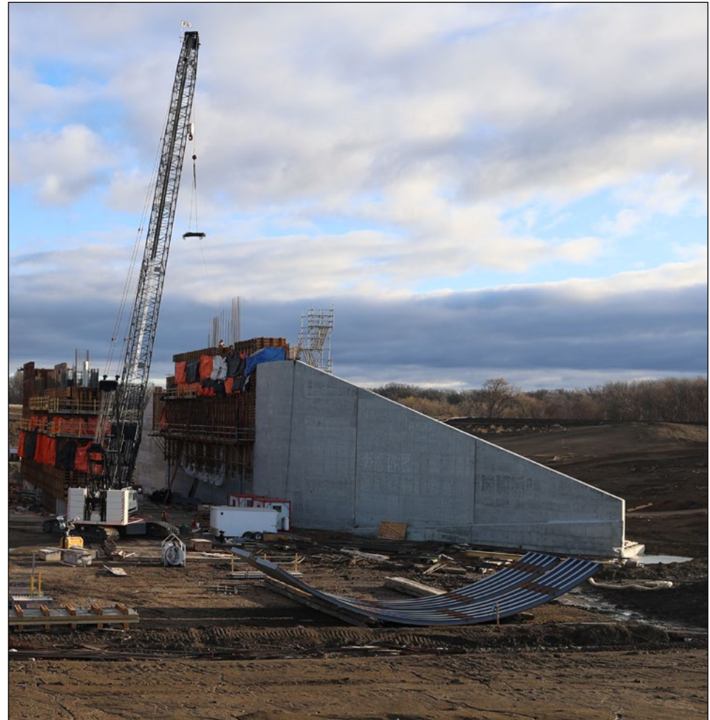
A skin plate delivery at the Red River Structure, seven miles south of Fargo, North Dakota and Moorhead, Minnesota, April 18. USACE St. Paul District photo by Melanie Peterson
